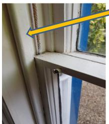
Staff bead should be installed so that the sash window can slide but there is not so much play as to allow draughts.
