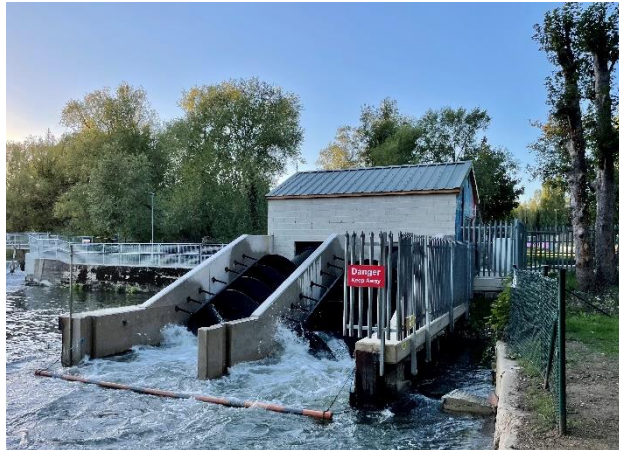
Figure 1: the new Reading Hydro turbines
